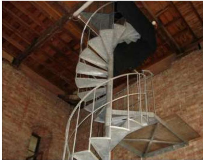
**Figure 1. The new spiral staircase, which replaced the old wooden ladder**
